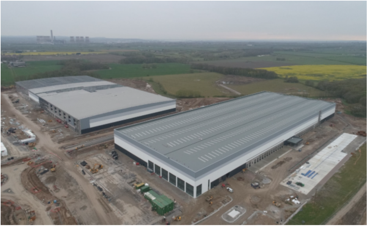
Application site (Unit 2 Foreground, Unit 3 Background)
