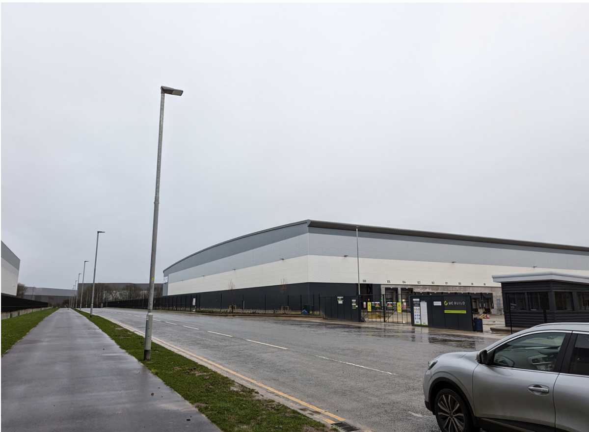
Access road to Unit 4. Unit 3 shown.
