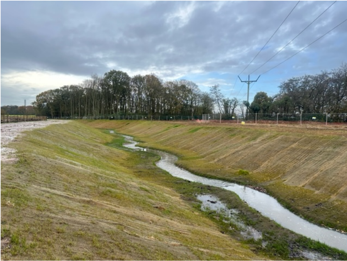
Further views of river diversion works.
