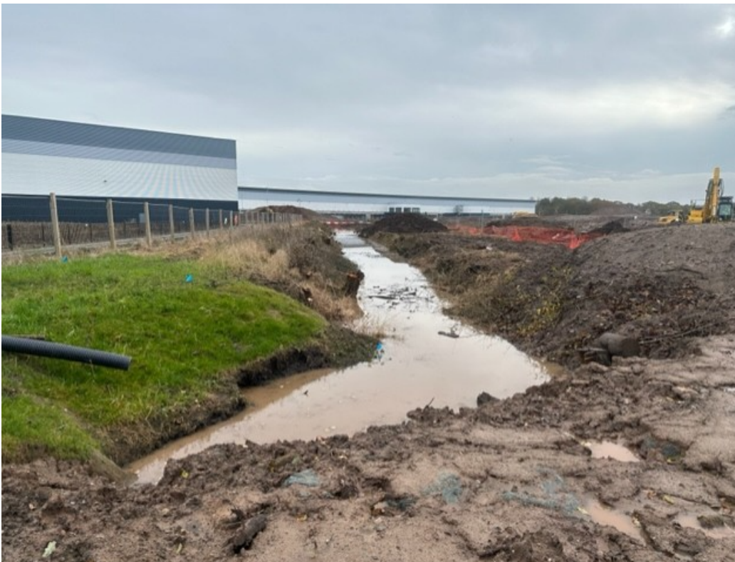
View towards plot of Unit 4 before completion of the river diversion
